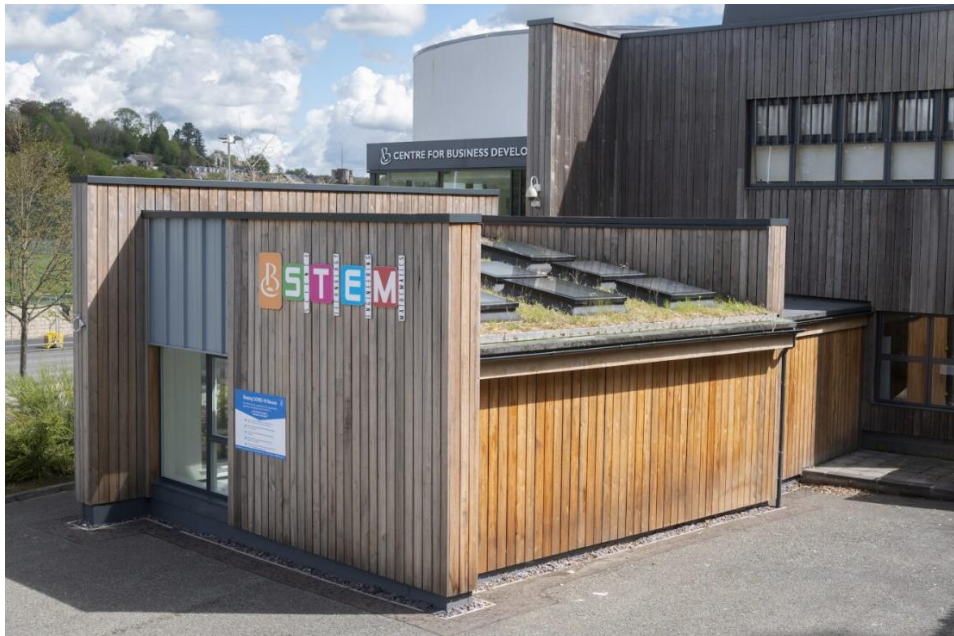
Figure 9: The Borders College STEM Hub Eco Room, based in Hawick, utilises a Passive House approach to ensure high-energy efficiency, making the best use of new materials, super insulation, triple glazing, solar gain and a green roof (Credit: Borders College, Eco Room news article ).
