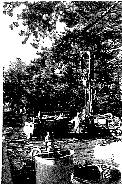
Geothermal, Red Hill
